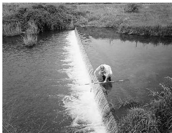
Fig. 4. A weir (drop) at the Fushino River in Yamaguchi Prefecture before the construction of “Mizube-no-Kowaza” fishway.
