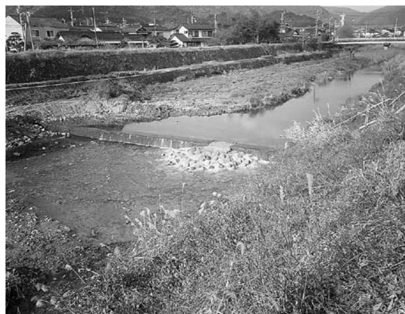
Fig. 5. “Mizube-no-Kowaza” fishway constructed to the Fushino River.
