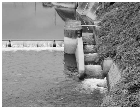
Fig. 9. Movable weirs with fishway at the Asa River in Yamaguchi Prefecture before the construction of "Mizube-no-Kowaza" fishway.
