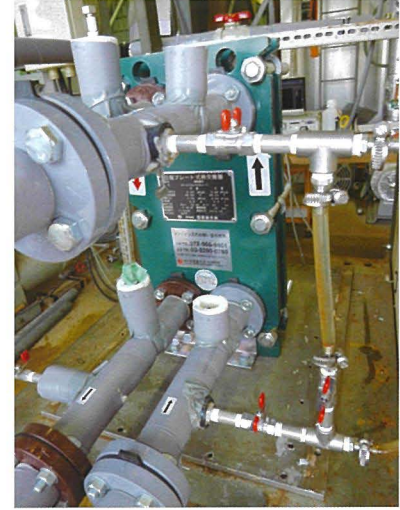
Fig.3 Test heat exchanger (Plate type)
